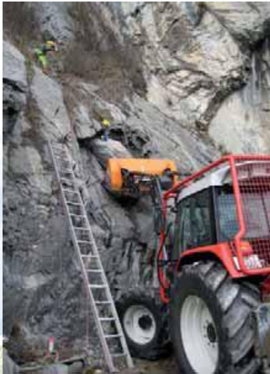
Positioning the Test Block
