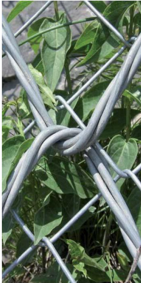
Mesh to Mesh Connection - Single Twist
